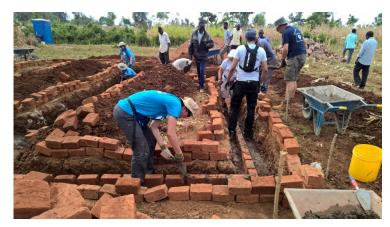
After the introductions we got to building. The materials were already on site and the builders had dug trenches and layed concrete, so our first job was mixing mortar with spades and ferrying bricks. The experienced builders on our team and localy hired ones, positioned the bricks and we filled in the gaps and put mortar on top.
