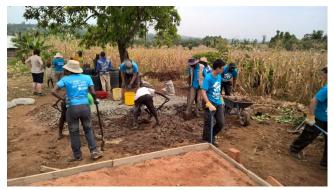
barrows of dirt then we mixed a ginormous batch of concrete and barrowed it onto the plastic. The recipe was nine bags of cement each one weighing about a small adult. Then came forty barrows of aggregate (gravel) and forty barrows of sand, along with two bathtubs worth of water. This was then mixed in a pit in the ground with spades.
