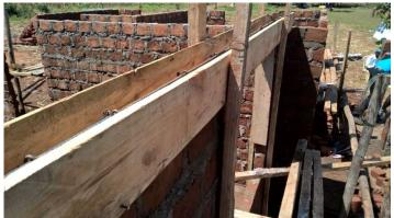
We wound metal wire round metal poles to create the ring bar that went on top of the walls. Either side, the builders nailed planks. The concrete would be poured into the trench and set around the metal that would strengthen it. This concrete ring bar would then support the roof.
